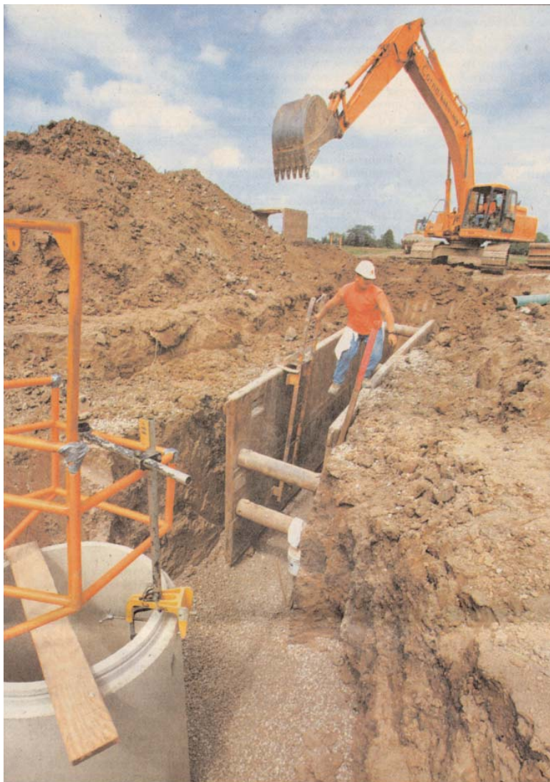
FRED SQUILLANTE | DISPATCH Albert Breech is part of a crew installing sanitary sewers in the Walker Meadows development in Union County.
